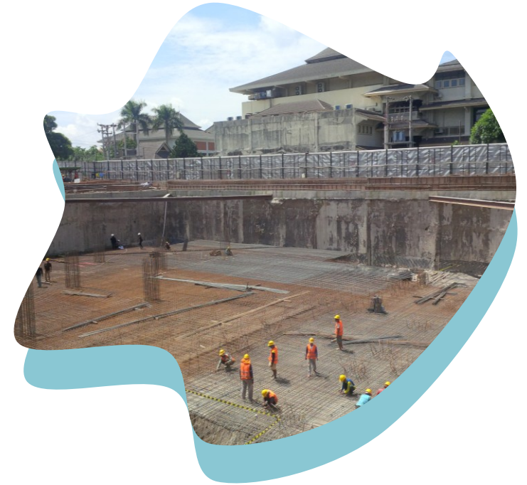
DIAPHRAGM WALL (cast in situ) CWS System
