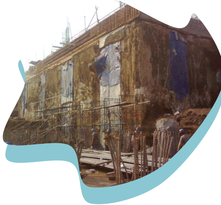
DIAPHRAGM WALL (cast in situ) CONTINUOUS SYSTEM
