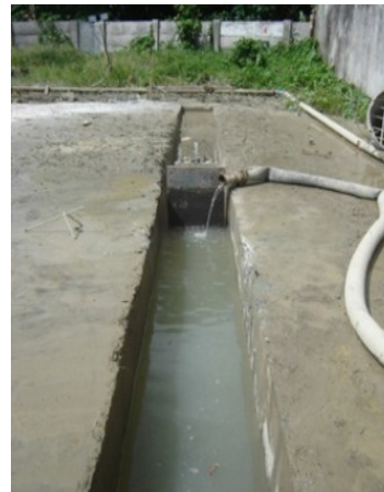
Pengisian Slurry stabilizer
