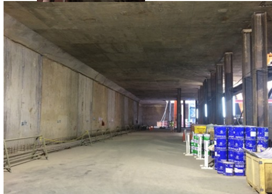
DW (continuous system)
