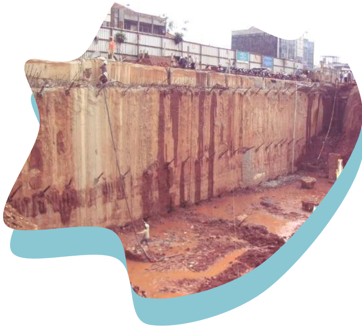
DIAPHRAGM WALL (cast in situ) CWS SYSTEM
