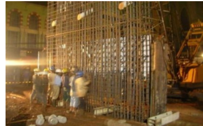
Install keranjang besi
