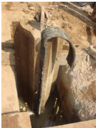
Install CWS Joint + rubber waterstop
