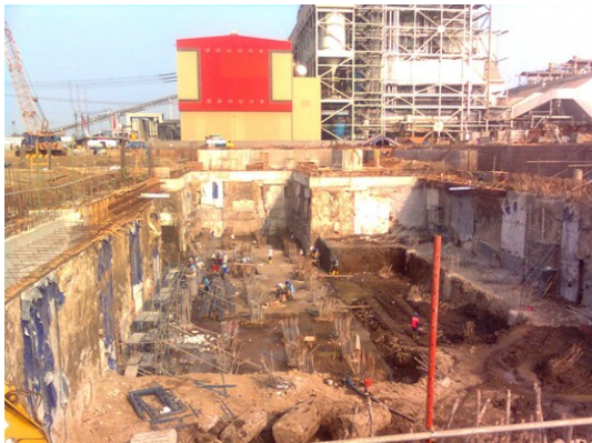
DW (continuous system)
